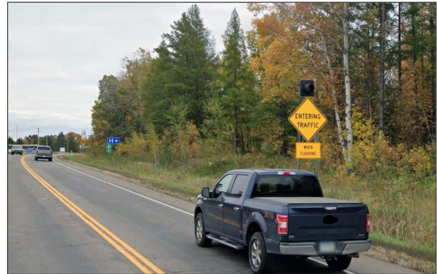
Figure 25. Photo. Intersection conflict warning system.
