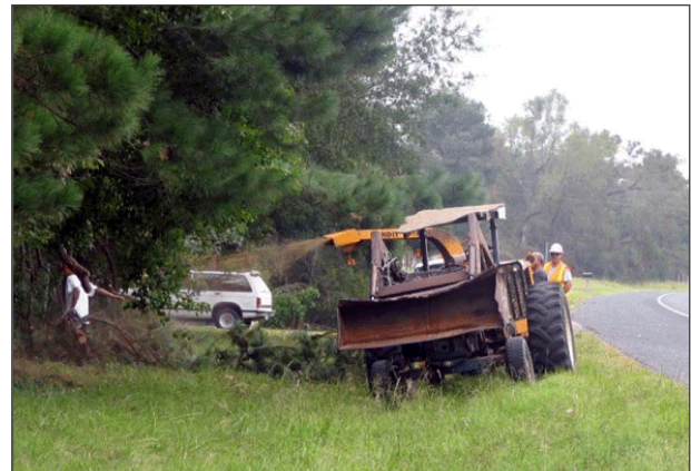
Figure 20. Photo. Maintaining a clear zone outside a curve.
