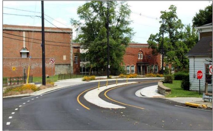
Figure 56. Photo. Mountable median with a traffic calming effect along the horizontal curve at the base of the steep downgrade.
