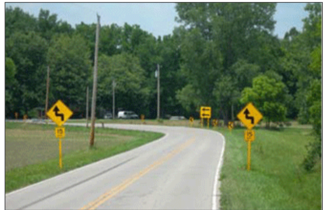
Figure 14. Photo. Enhanced curve signing (doubled signs and retroreflective posts).
