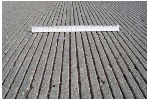
Figure 35. Photo. Transverse grooving on concrete pavement.
