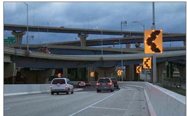
Figure 22. Photo. Sequential dynamic curve warning system.
