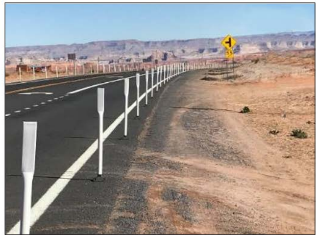
B. Narrowed 5-foot shoulder comprised of 2 feet of paved shoulder and 3 feet of stabilized shoulder.
