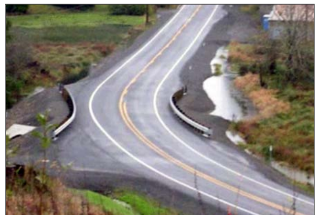
Figure 17. Photo. Lane and shoulder widening through horizontal curve.
