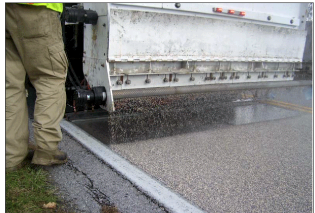
Figure 16. Photo. Calcined bauxite aggregate applied to polymer adhesive.
