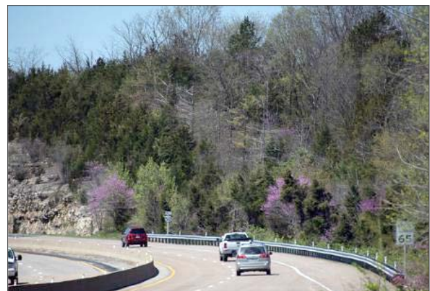
Figure 21. Photo. Longitudinal barrier shielding outside of curve.
