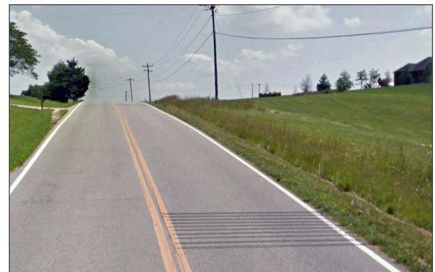
Figure 24. Photo. Transverse rumble strip warning of intersection beyond crest vertical curve.
