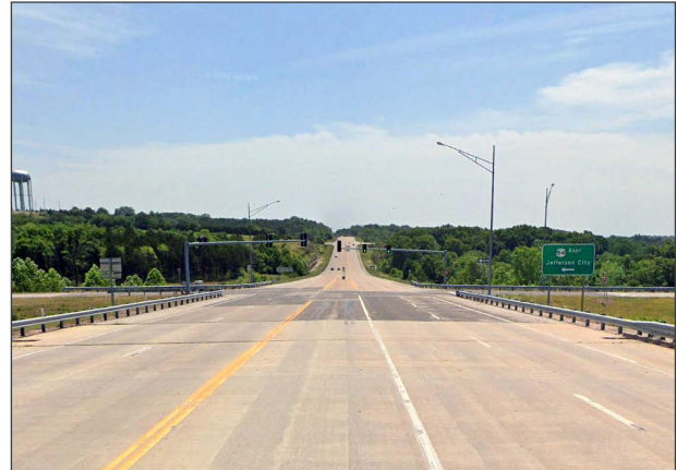
Figure 27. Photo. High friction surface treatment on tangent section in advance of signal on steep downgrade.
