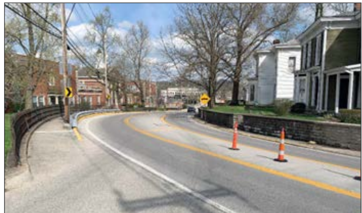
Figure 57. Photo. Retaining walls affect sight distance, but moving them would create disruption to the built environment and require investment because of the homes, businesses, and trees behind the walls.
