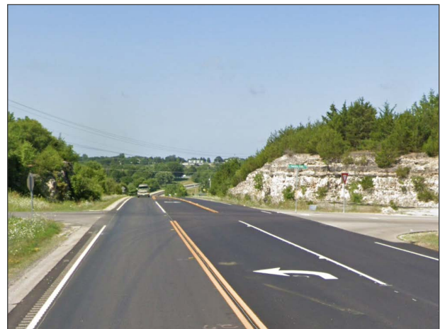
Figure 26. Photo. Dedicated left-turn lane on rural two-lane roadway.
