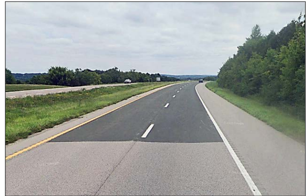
Figure 36. Photo. High friction surface treatment to reduce wet weather crashes.
