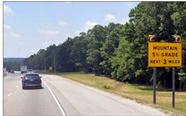
Figure 29. Photo. Grade warning sign with supplemental flashing beacons.
