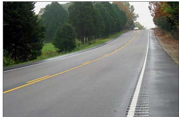
Figure 28. Photo. Widened and paved shoulder improvements.
